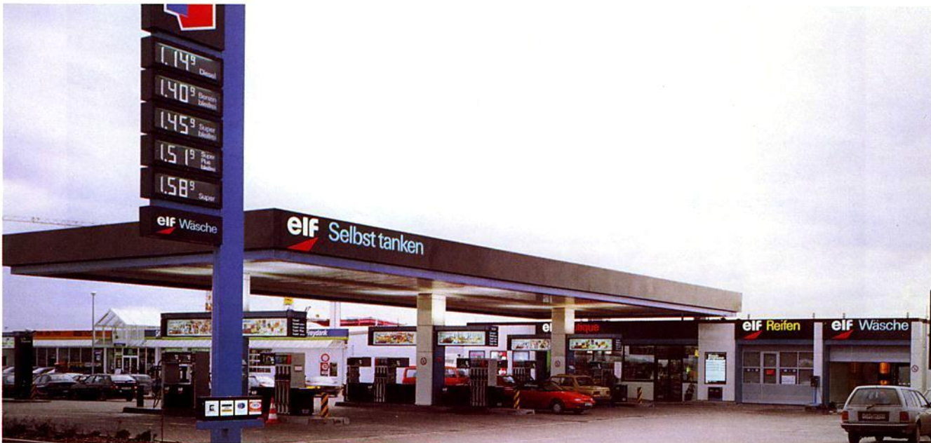
The AWAS petrol station concept: fuel pumps, workshop, roll over wash and self service bays are all drained via the AWAS-RC system and one AWAS-HI-2000 separator. An AWAS-FLOT-B recycles car wash water
